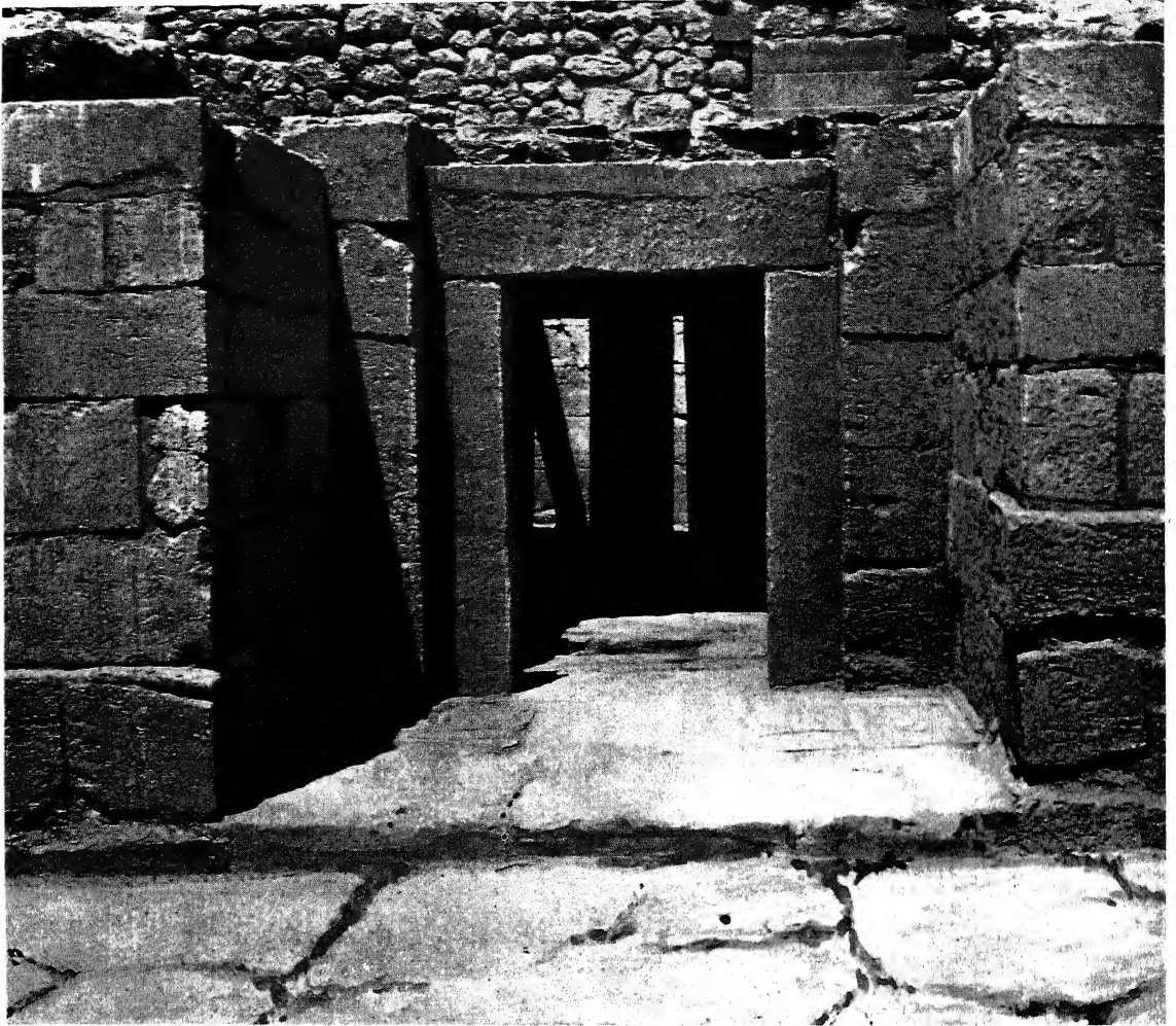
FIG. 948. WALLED BAY OF BASEMENT PORTAL, LEADING TO ENTRANCE HALL.
